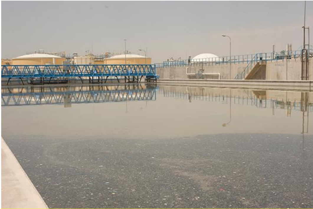
Jordan, As Samra wastewater treatment plant. Image courtesy of GDF SUEZ / ABACAPRESS / Lyons Bill.
